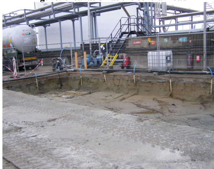
Figure: excavation at the central road
