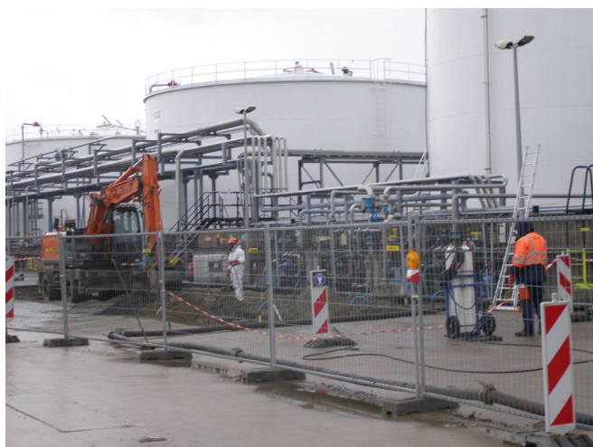
Photo: Excavation works and risk zone perimeter
