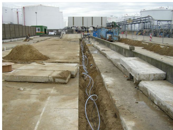
Photo: Installation of piping in grooves
