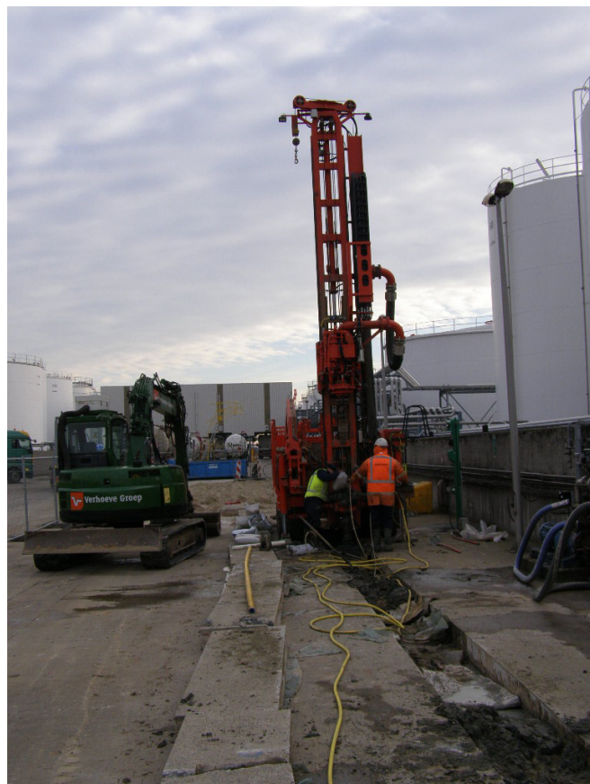
Photo: Installation of injection and extraction wells
