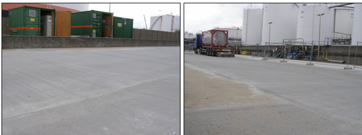
Figure 3. Photos of renewed concrete cover in the midway area.
